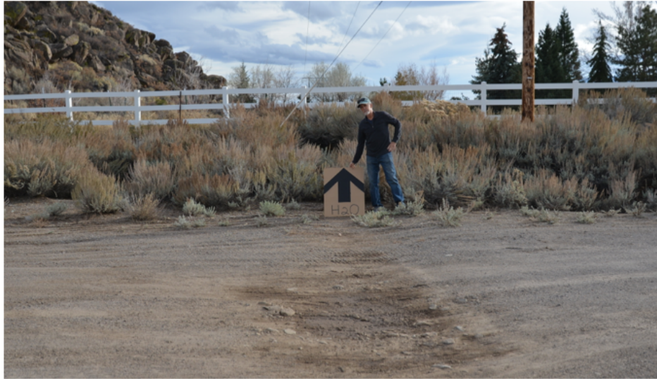
Ascente storm water flow path across private driveway
