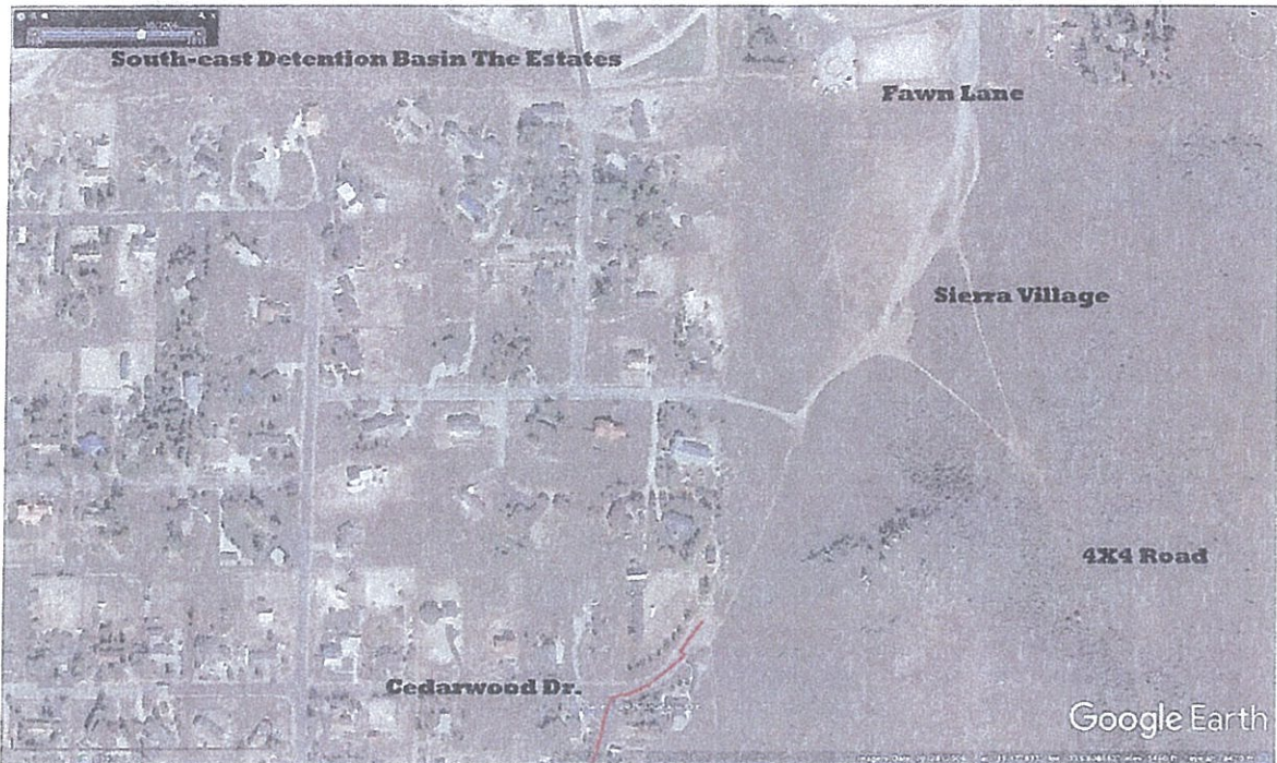
Goggle Earth image November 2006. Note the cleared vegetation and compaction in the flats south of Fawn Lane. Also the Detention basin in the Estates is nearly full of storm water.
