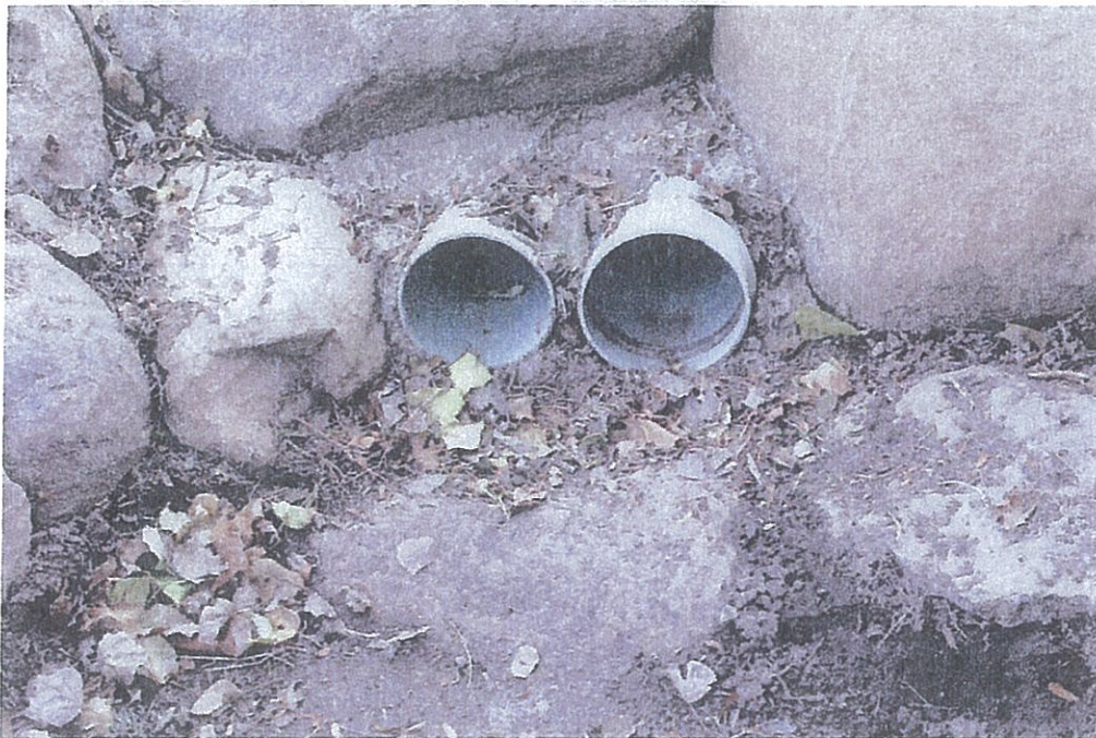
P6 Additional plumbing for storm water on private property.
