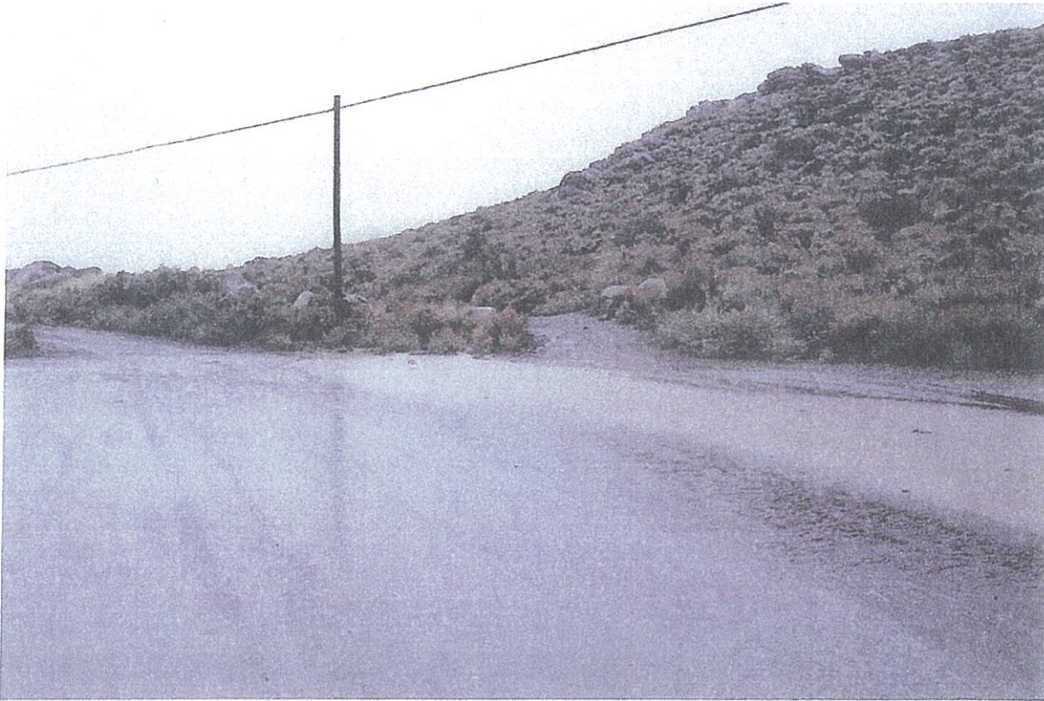
Storm water runoff from area of Sierra Village onto Cedarwood Drive October 16, 2016 5:39 PM.
