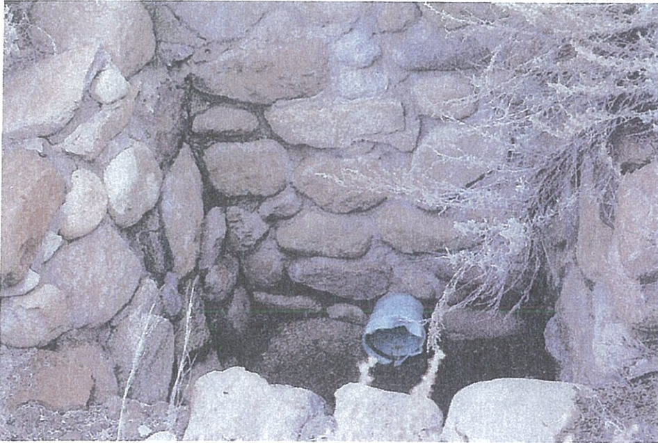
P4. Storm water path under private property, pipe size 9".
