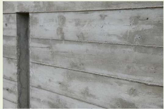
Board Formed Concrete
